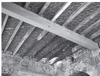
View of Madras terrace roof under construction
