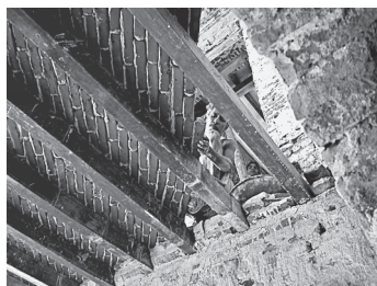
View of Madras terrace roof under construction
